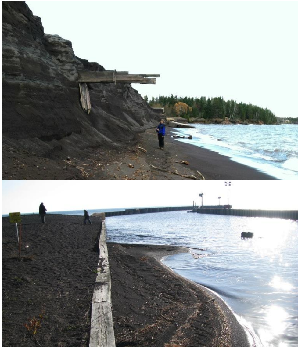
Figure 4. Stamp sands erode from the enormous tailing pile at (Above) Gay and over-top the (Below) Traverse River Seawall, spilling into the Traverse River channel.
