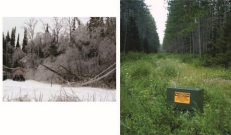
Power Line retrofit/burial
